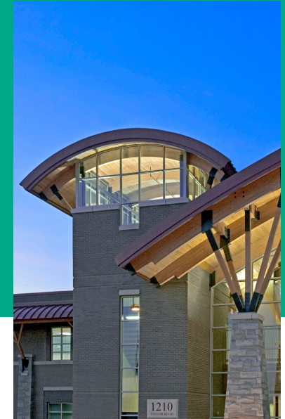
Exposed timber brackets that support deep roof overhangs give a vigorous profile to the curved roofs at the entrance and atop the stair tower.
